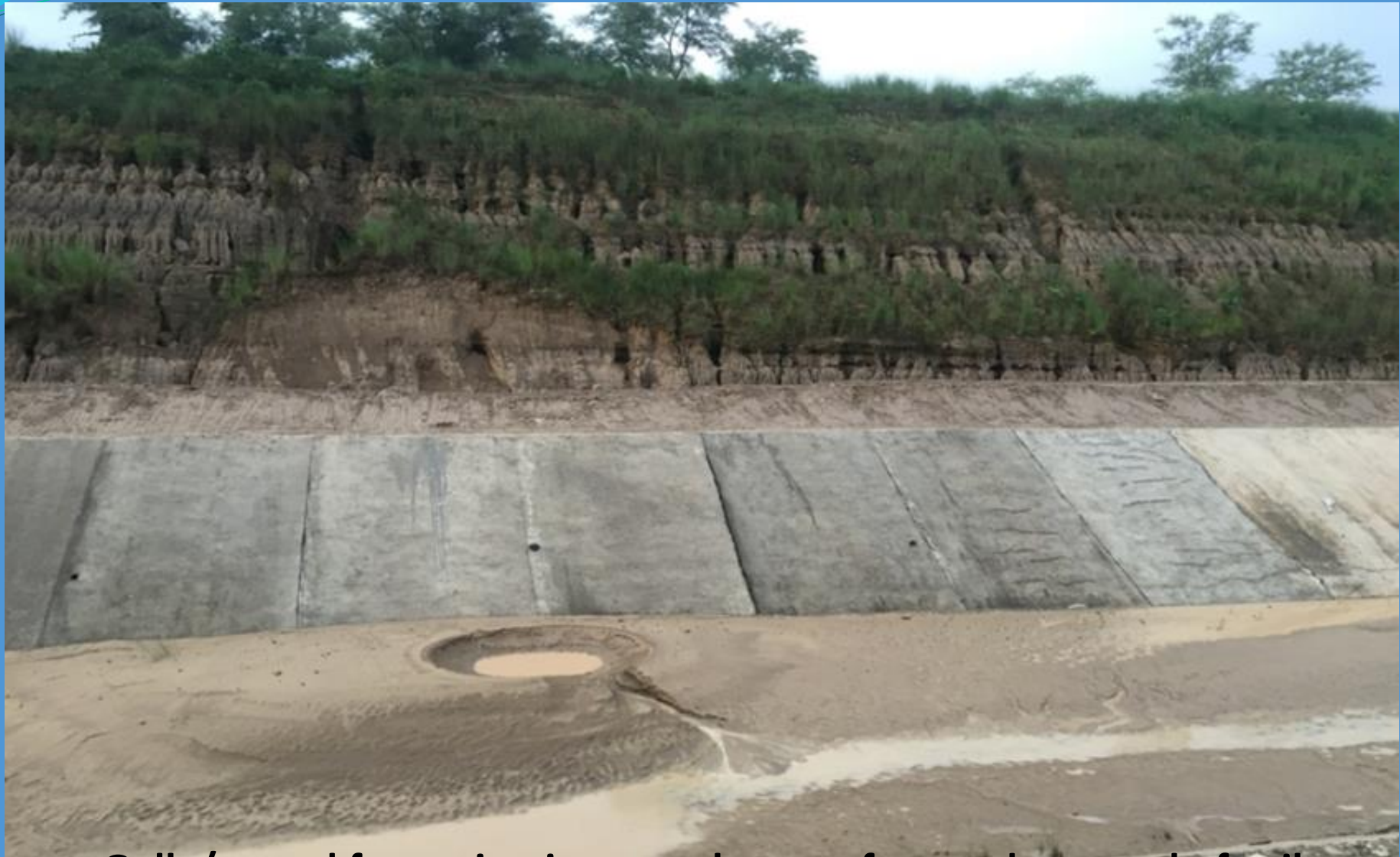
Gully/tunnel formation in natural cut surface and removal of soil
