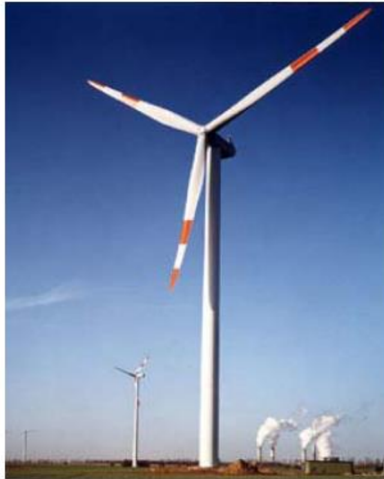
Prototype of 80 m tall Nordex 2,5 MW wind turbine located in Grevenbroich, Germany (Danish Wind Industry Association)
